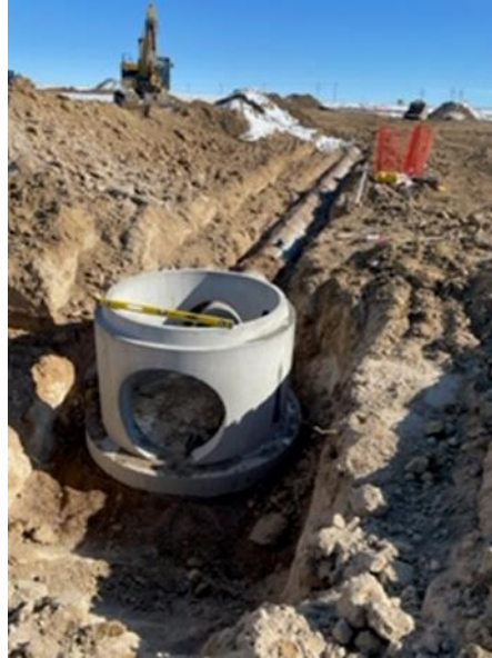
Inspection of storm Pipe at Pautler Farms
